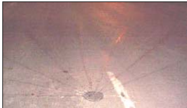
Spray Nozzle in Pavement
